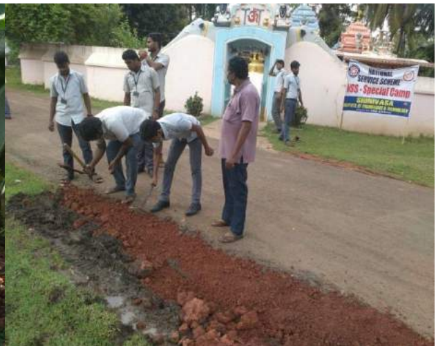
Figure 11 Road repair work.
