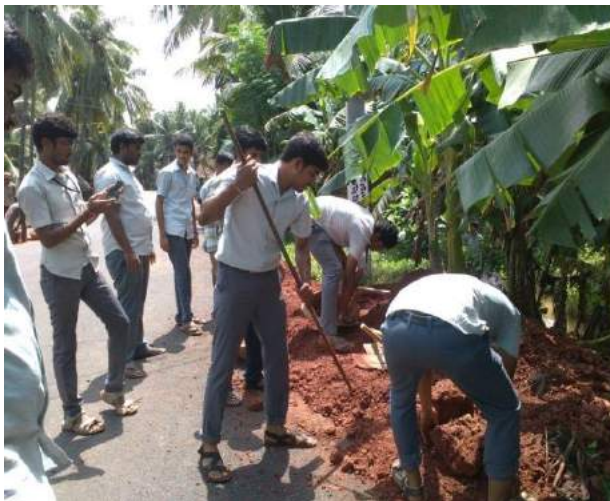
Figure 10 Road repair work.
