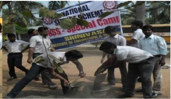
Figure 4 NSS Volunteers participated in Road Repair Work
