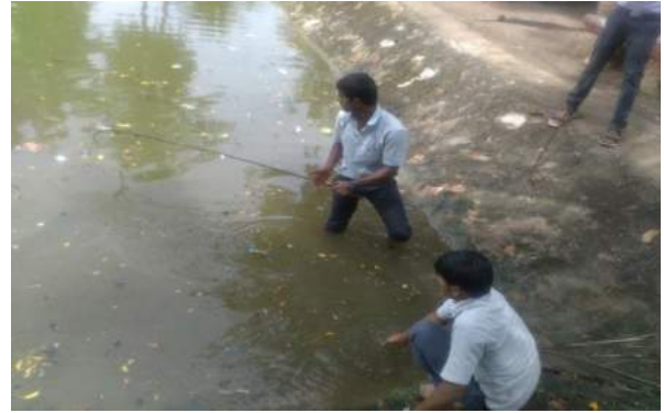
Figure 13 Water tank repair work
