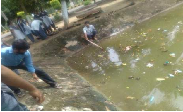
Figure 12 Water tank repair work
